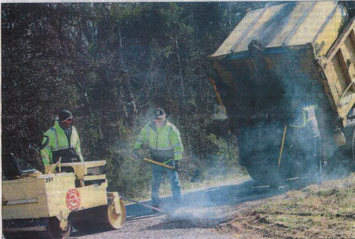
A Wilson County Road Commission crew works to fill a pothole on Long Oak Road in Gladeville on Tuesday afternoon. Pictured are (from left) Bryan Graves, Gary Heird and Glenn Coggins.
